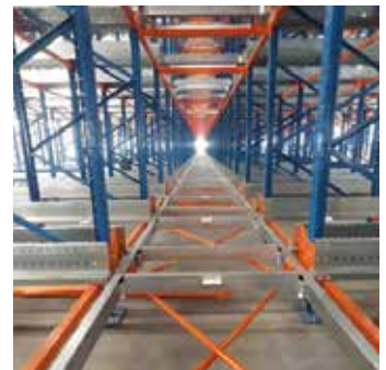
3) 4-Ways Shuttle System that suite perfectly for medium-rise warehouses and building for high density storage as well. This system installed rails within the racking system to allow the shuttle cart move horizontally along the racking system for storing and retrieval of stored pallets, containers within the racking system. This has resulted in another level of work efficiency and storage automation into ones operation storage space for goods.
