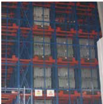
3) 4-Ways Shuttle System that suite perfectly for medium-rise warehouses and building for high density storage as well. This system installed rails within the racking system to allow the shuttle cart move horizontally along the racking system for storing and retrieval of stored pallets, containers within the racking system. This has resulted in another level of work efficiency and storage automation into ones operation storage space for goods.
